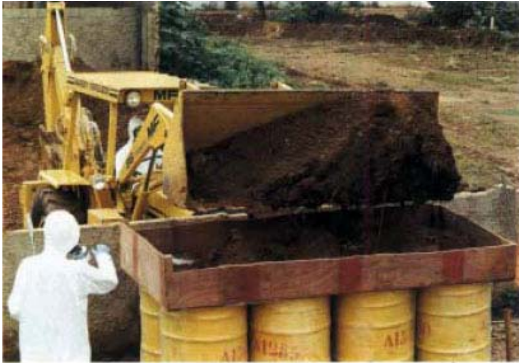
18. An improvised way of filling eight drums simultaneously with contaminated soil.
