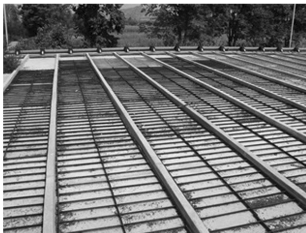
Fig. 4 The large-scale cultivation plant with a total area of 3000 m 2 made of concrete was constructed in Rupite, southwest Bulgaria. It consisted of thin-layer sloped platforms placed on the ground over which microalgae would flow. The platforms had a slope of 3% and were fitted with transversal baffles to increase culture turbulence
