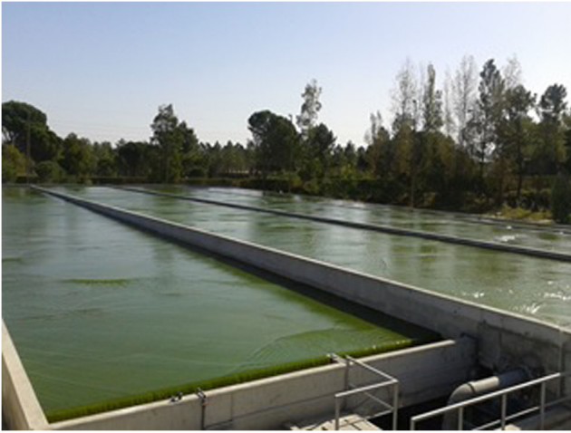
Fig. 13 A large-scale plant consisting of cascade raceway modules of 1500 m 2 (volume of 100,000 L) was installed in Pataias, Portugal, for the BIOFAT project (designed and built by the company A4F EU). The unit consists of two sloped platforms (declining of 0.5%), 10 m wide and 75 m long which form a cascade-like system running in opposite directions. This facility is a hybrid between a raceway pond and a sloping cascade since the layer thickness is about 40 mm, resulting in the S/V ratio of about 15 l/m. In this case, the operating biomass density is about 4 g/L DW (courtesy by Luis Costa)
